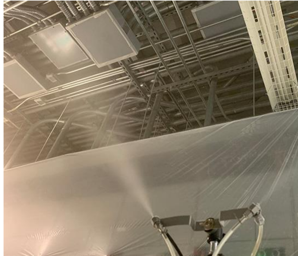
Sealing Air Leaks Behind Conduits While Protecting Control Panels
