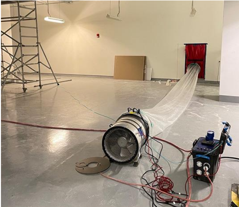
Pressurizing the Exterior Wall Cavity
