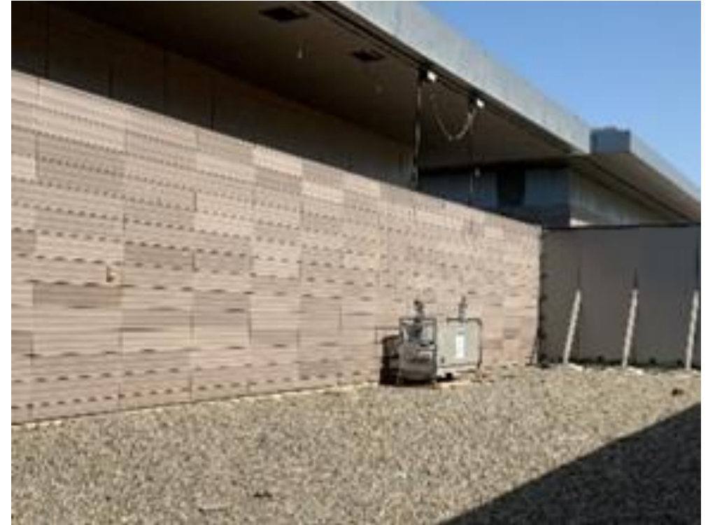
Exterior Wall at Mechanical Room
